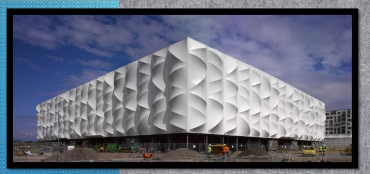
For the same games, Wilkinson-Eyre Architects designed a Basketball Arena in North London. The PVC wraps around a modular, easy-to-assemble steel portal frame. External walls are translucent, allowing daylighting in all the support spaces. Lighting can change color and intensity, creating interesting patterns.
