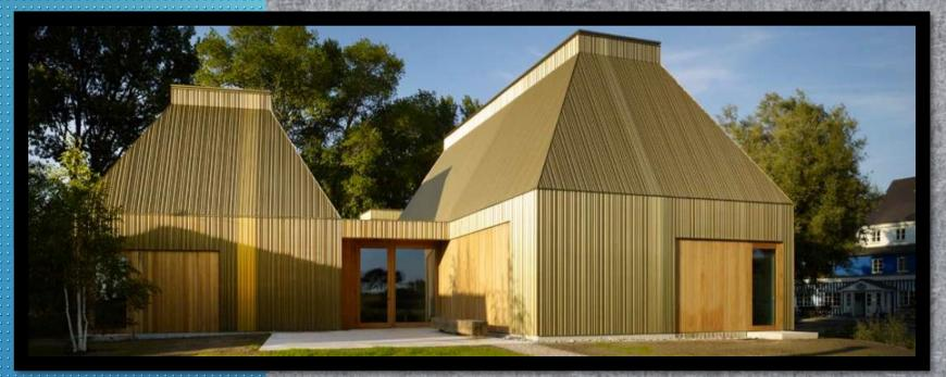
Staab Architekten designed the new (2013) Ahrenshoop Museum of Art as a sculpture clad in brass. The exterior material is a specialty metal, a TECU brass manufactured with a "welltec" process allowing edges and bends configurable both in the factory and on site.
