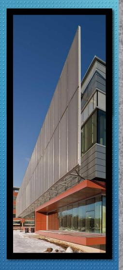
Canmet Material's 2015 main facility in Hamilton, Ontario by Diamond Schmitt Architects has a dual-envelope for passive solar shading. Its lightweight, insulating, structural KALWALL panels allow glare-free natural daylight, ultimately reducing energy use and thus greenhouse gas production.
