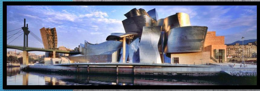
Frank Gehry is well-versed in titanium, stainless steel, and numerous other modern metals. This is the pinnacle of his design oeuvre, the Guggenheim Museum Bilbao in the Basque region of Spain. The titanium panels curve and torque in all planes, and are met with glass and limestone cladding at the base. The exterior forms describe a bold, undulating, and forceful interior.
