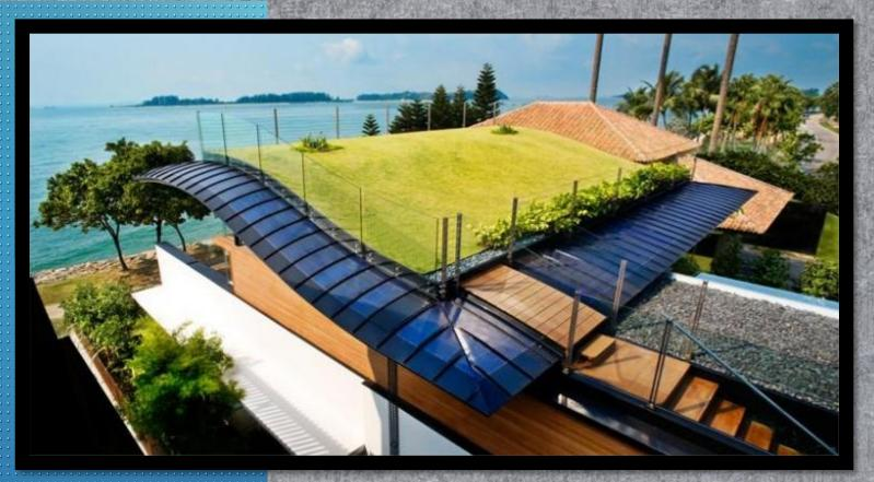
Guz Architects designed the Sky-Garden House in 2010 on Sentosa Island, Singapore. The home consists of a series of roof gardens, each providing the base for the level above. The photovoltaic panels at the top provide both energy and solar shading.
