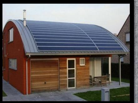
Building-Integrated Photovoltaics are the latest trend in alternative energy. The top two images show a home with a tin oxide film coating in lieu of separate panels. Below is an entire community in Germany that produces more energy via solar than it uses.
