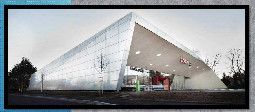
Love Architects designed this 2012 Austrian supermarket to produce more energy than it uses. The building façade consists of panels of galvanized sheet steel, and contrasting wood. The steel composes the outer seal of a highly-insulated building envelope, containing ventilation, heatrecovery and daylight control systems.
