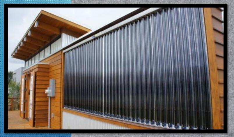
Students from the University of Maryland assembled a 2011 award-winning Solar Decathlon house with passive solar orientation, photovoltaics on the butterflyshaped roof, and solar thermal panels on the south-facing side, providing hot water.
