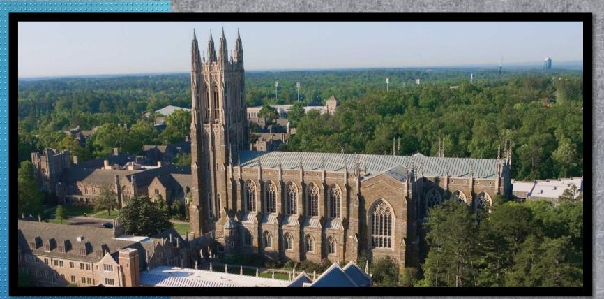
Architect Julian Abele designed the Duke University chapel in Collegiate Gothic style from 1930-1932. The lead-coated copper roofing panels were removed and replaced in 2015, while crews repaired joints in the limestone mortar ceiling.
