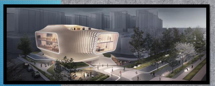
DIA Studio in Amsterdam produced this solution for the Daegu Gosan Public Library in South Korea, with its volume wrapped in a PVC membrane, pre-manufactured and inexpensive. The material is both frame, providing structural support, and tensile membrane, providing a building skin. The translucency of the material creates an interesting display at night.
