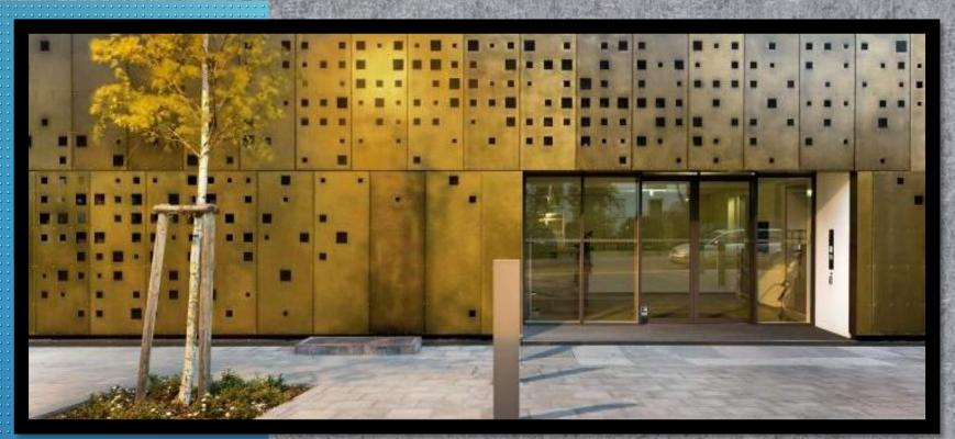
JSWD Architekten of Koln, Germany designed the Adaptronik Transfercenter at the Fraunhofer Institute in Darmstadt in 2012. The façade is made of sandwich plates of brass, which mechanically adapt and move, continually updating the building elevation.
