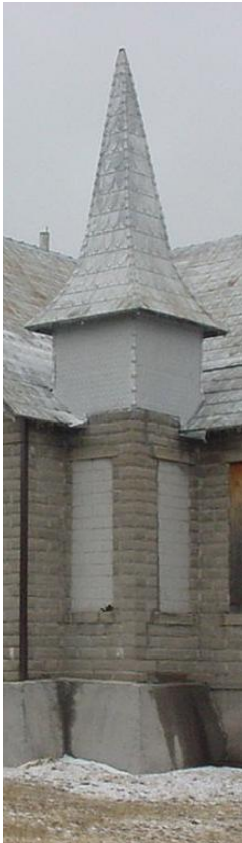
Left: Steeple at northwest corner. Note fully intact spire and later angled concrete buttress at base.
