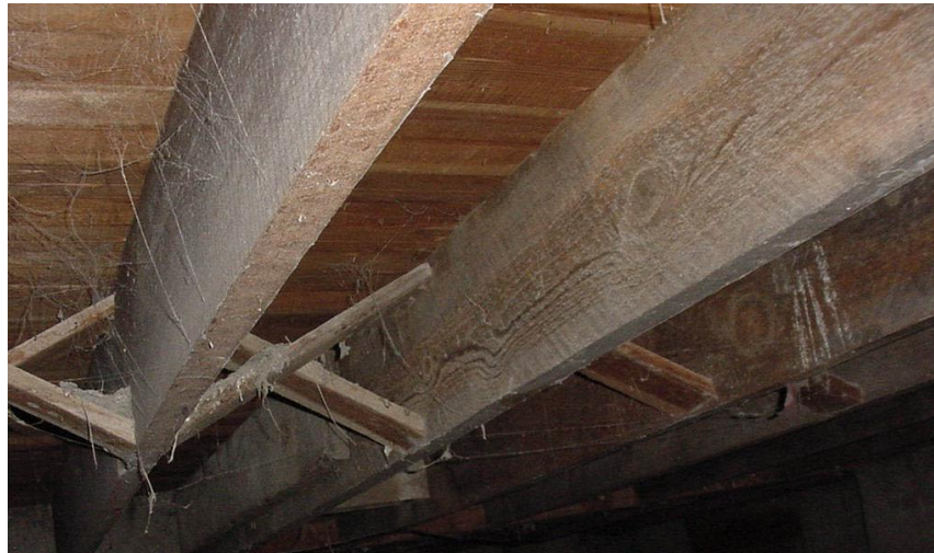
Main floor framing joists and cross bridging.
