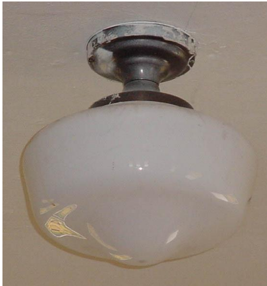
Left: Pendant light fixture in sanctuary.
