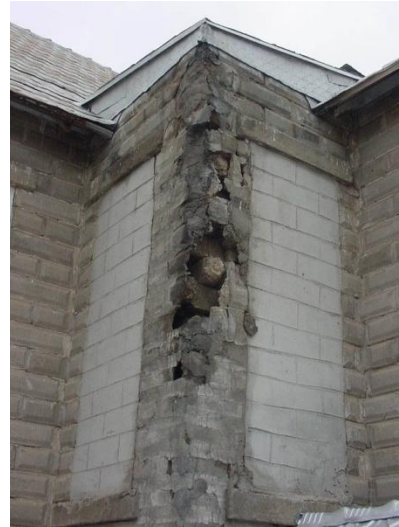
Southwest steeple detail.
