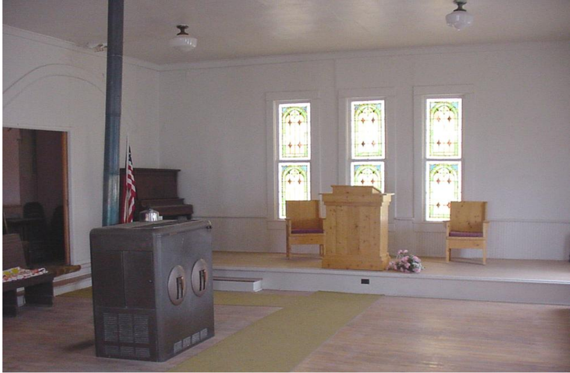
View of sanctuary looking north. Note wood arch at west wall, hardwood flooring, wood dais platform, plaster walls and ceiling, and wood bead board wainscot.
