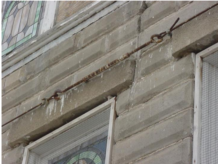
Turnbuckle at north elevation face.
