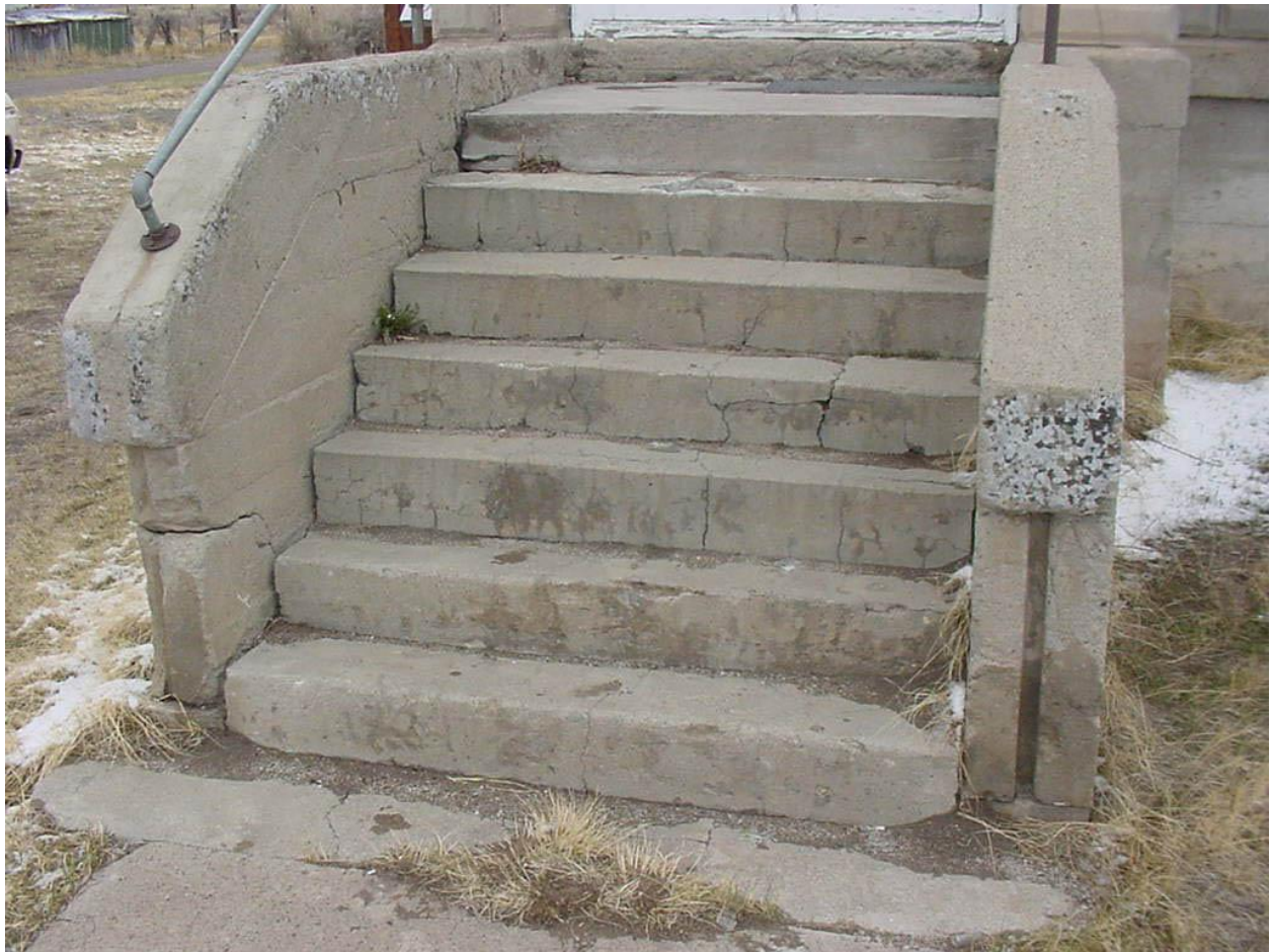
Main entry concrete stoop.
