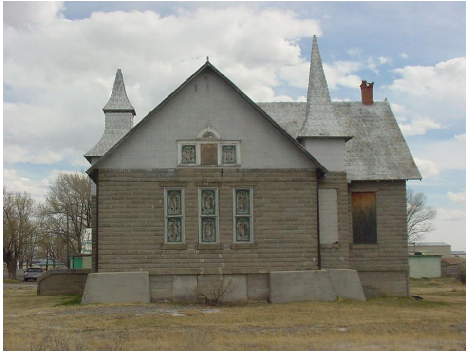
Side (north) elevation. Note buttresses at corners.
