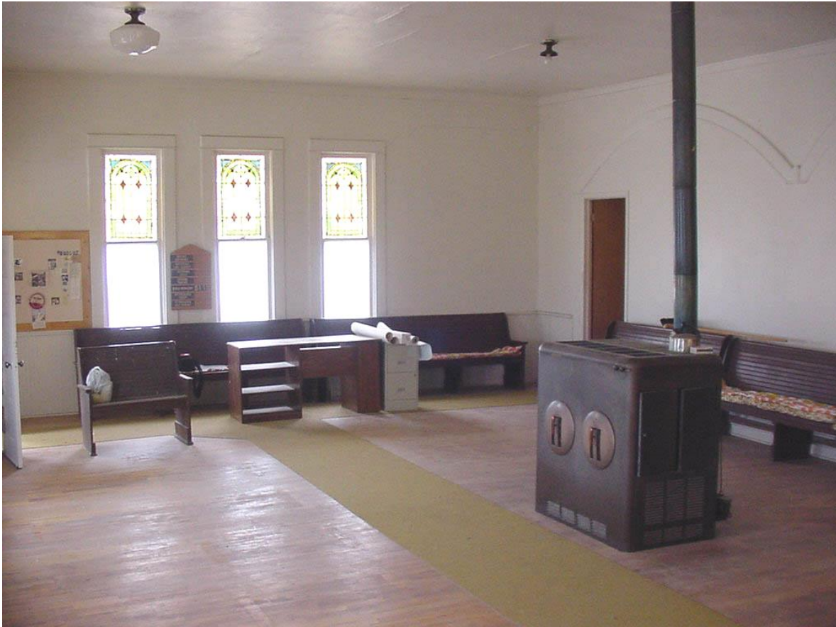
View of sanctuary looking south. Note wood arch at west wall, hardwood flooring, plaster walls and ceiling, and wood bead board wainscot.
