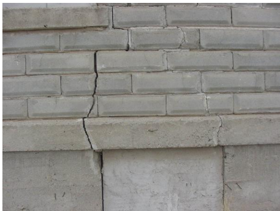
Exterior plinth and cracked masonry above.
