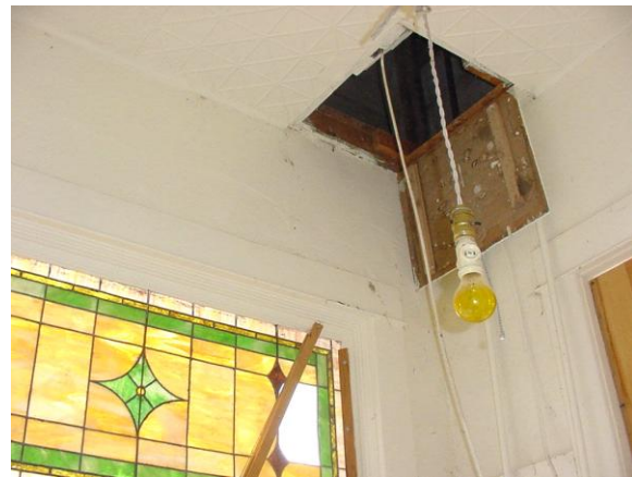
Tin ceiling (and belfry hatch) in vestibule.
