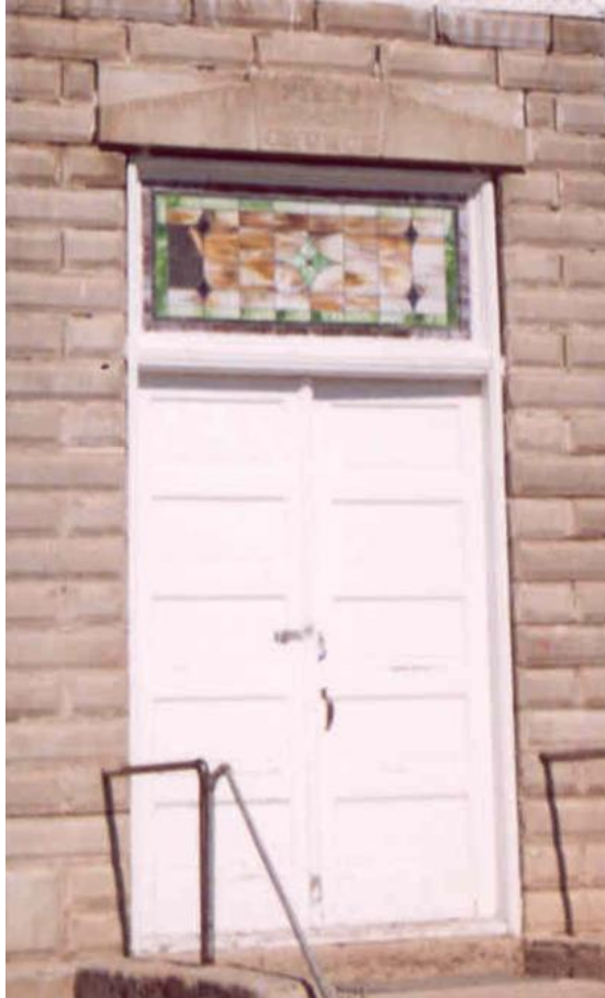
Main entry doors.
