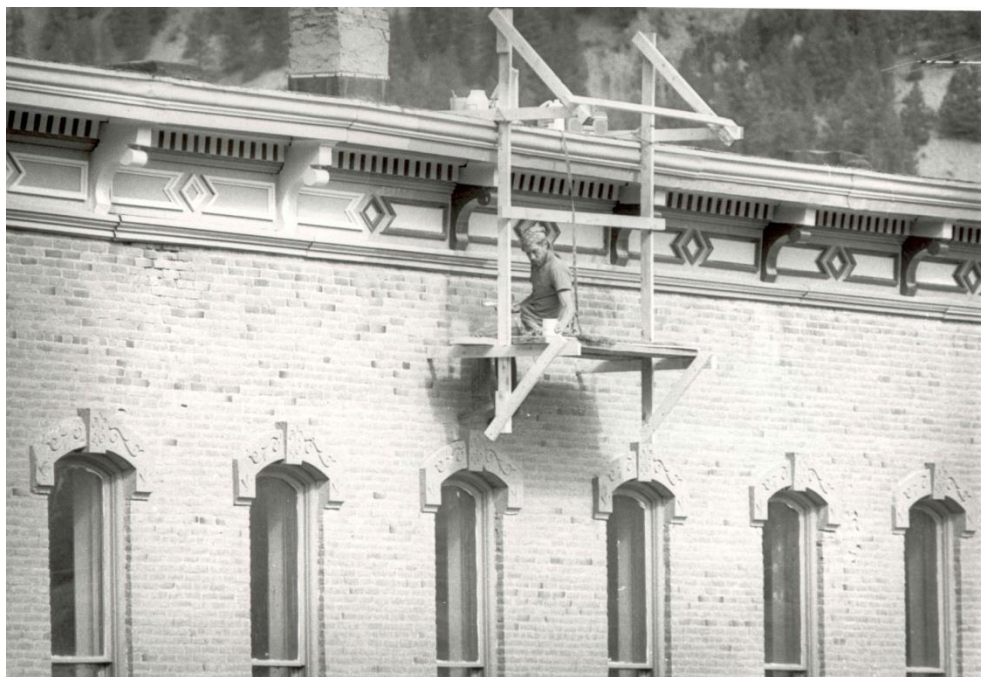
Cornice painting with makeshift scaffold. Photograph circa 1987.
