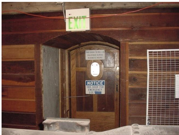
Lower level at exit door.
