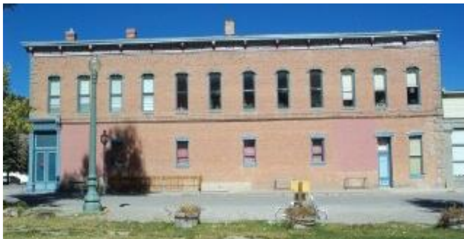
Hough Building South Elevation
