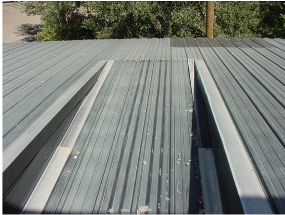
Metal seam roof at second level.
