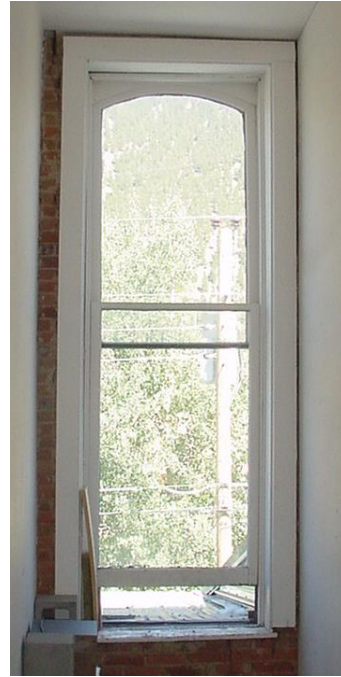
Upper level window.
