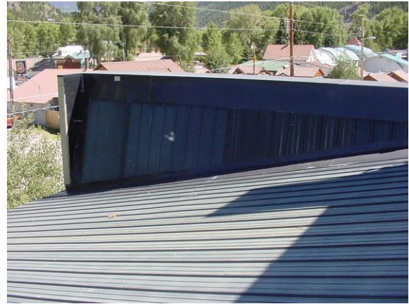
Metal seam roof, looking south.
