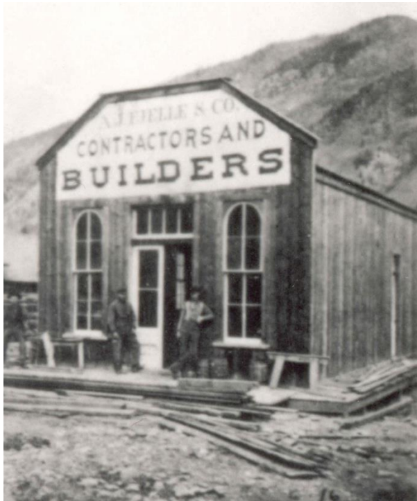
A. J. Fielle & Company Contractors and Builders
