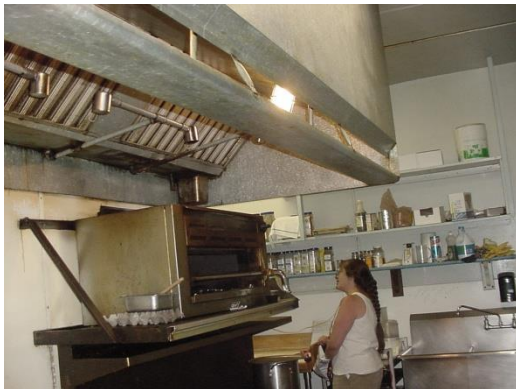
Kitchen, looking east.
