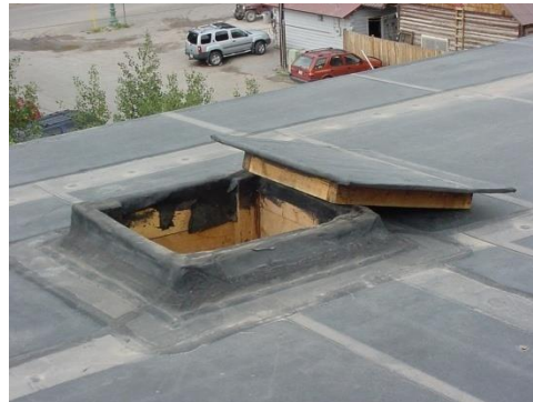
Detail at east roof hatch.
