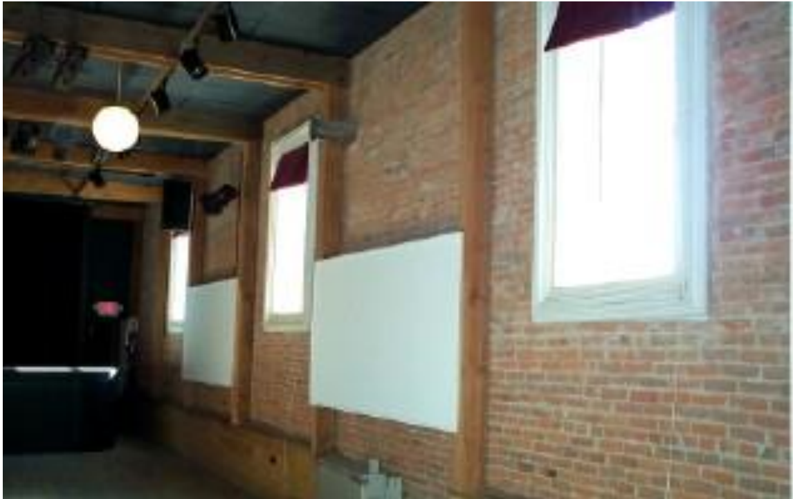
Above: Windows on south wall of theatre.
