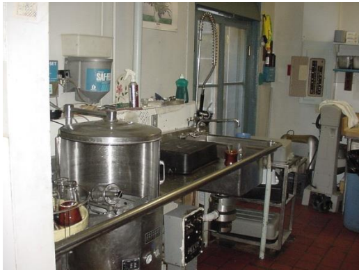
North wall of kitchen.
