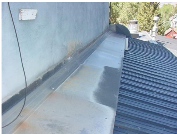
Sheet metal flashing at metal roof
