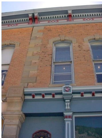
Cornice and upper cornice.
