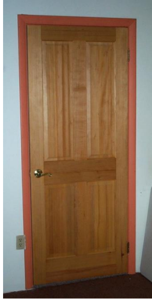
Non-original main level restroom door Wood, four panel.
