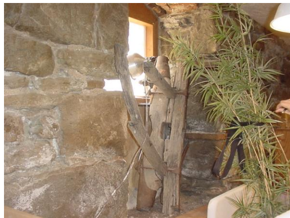
Lower level stone wall with lightwell.
