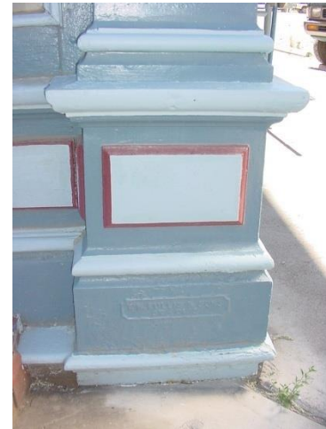
Cast iron storefront at building 1, and detail at pilaster base.
