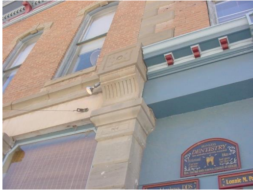
Cornice at building intersection.
