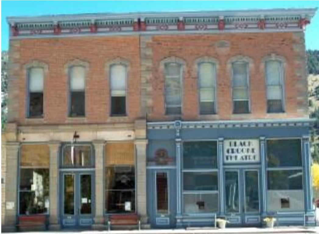
Hough Building West Elevation
