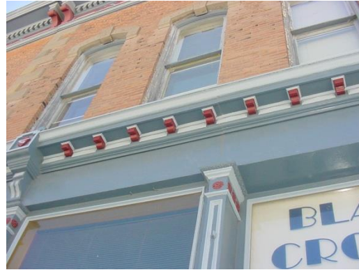
Cornice at building 1.
