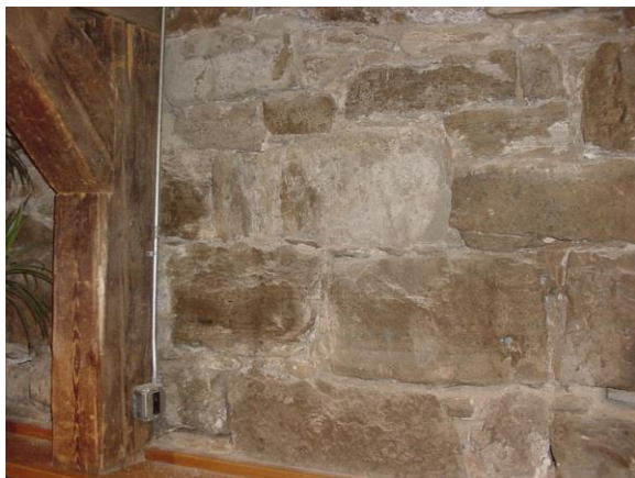
Lower level stone wall
