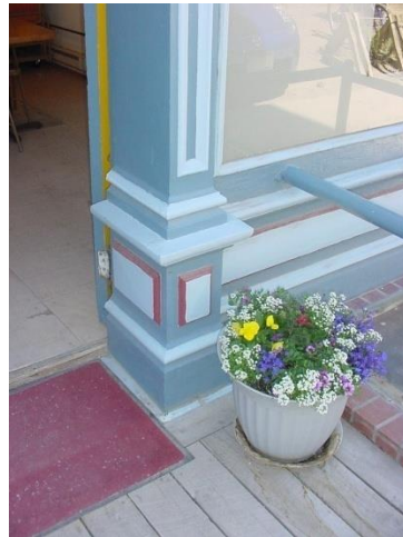
Cast iron storefront at building 1, and detail at pilaster base.
