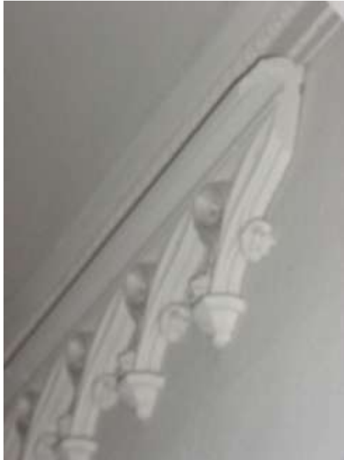
Left: Detail at terra cotta gothic cornice tracery.
