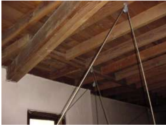
Ceiling framing beam and joists visible from fly loft.
