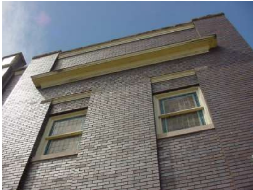
Typical view of wood cornice.
