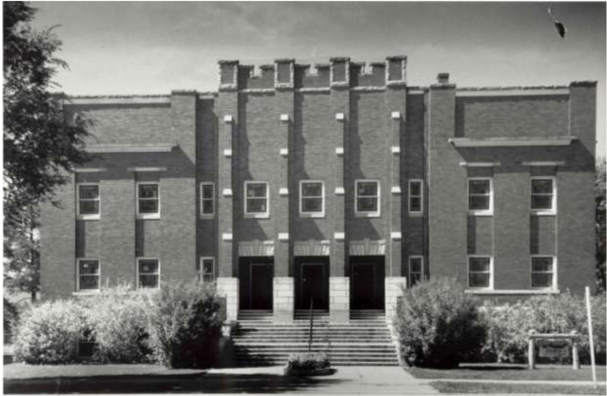
Front (East) Elevation, circa 1970. Photo prior to curvilinear ramp installation.
