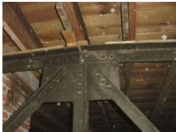
Detail at steel truss joint, with roof joists and decking above.
