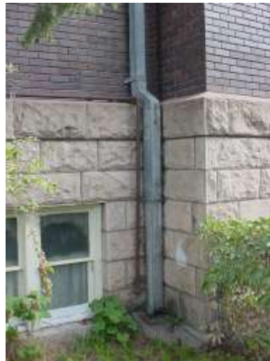
Leader at east side of south elevation.
