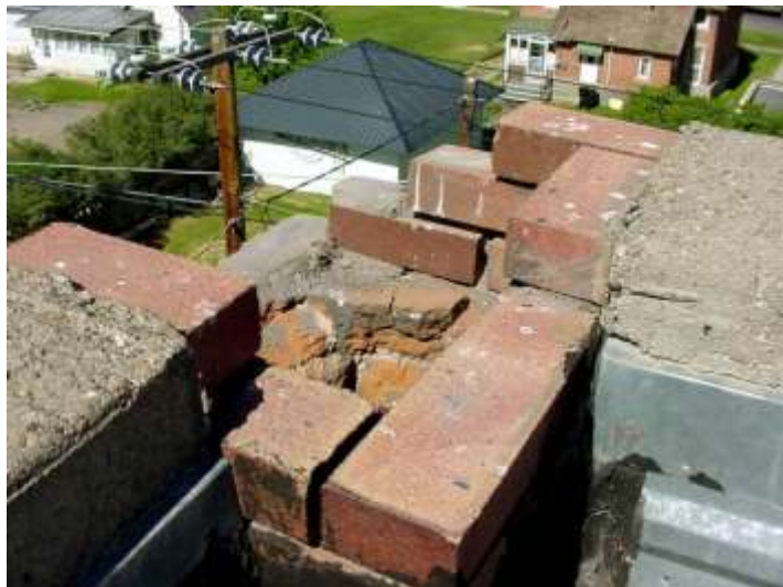
Chimney at southwest corner.
