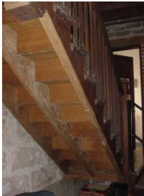
View beneath stair framing, showing wood stringers.
