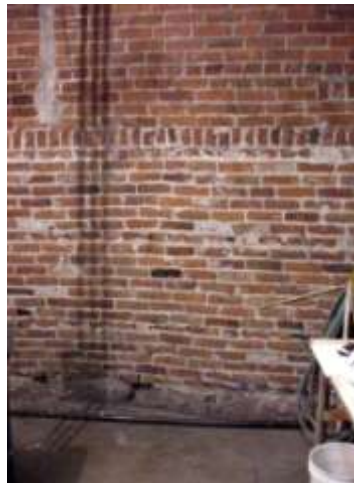
Interior masonry bearing wall in boiler room.
