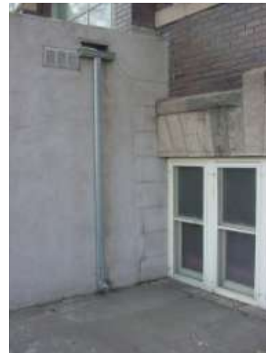
Scupper and leader at north entry vestibule.
