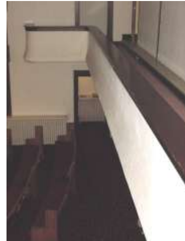
Mezzanine guardrail. (overlooking sanctuary)
