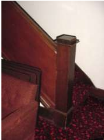
Mezzanine stair newel and handrail.
