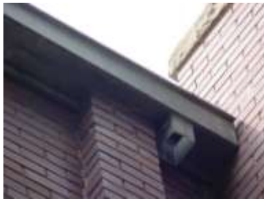
Gutter at west side of north elevation.
