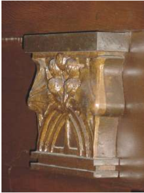
Left: Wood Corinthian capital Below: Detail of wood bracket at overhead partition.
