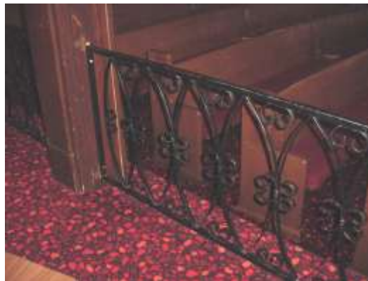
Railing beneath overhead door.
