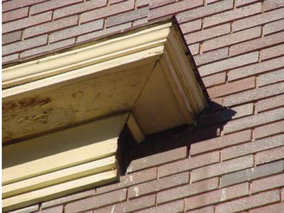
Above: Detail at cornice edge.
