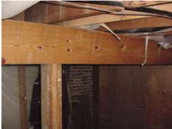
Composite beam in storage room below chancel. 2 x 12 joists below chancel.
