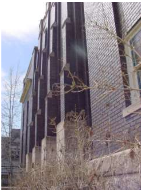
Left and right: Brick buttresses with smooth stone bases and stone amortizements.
