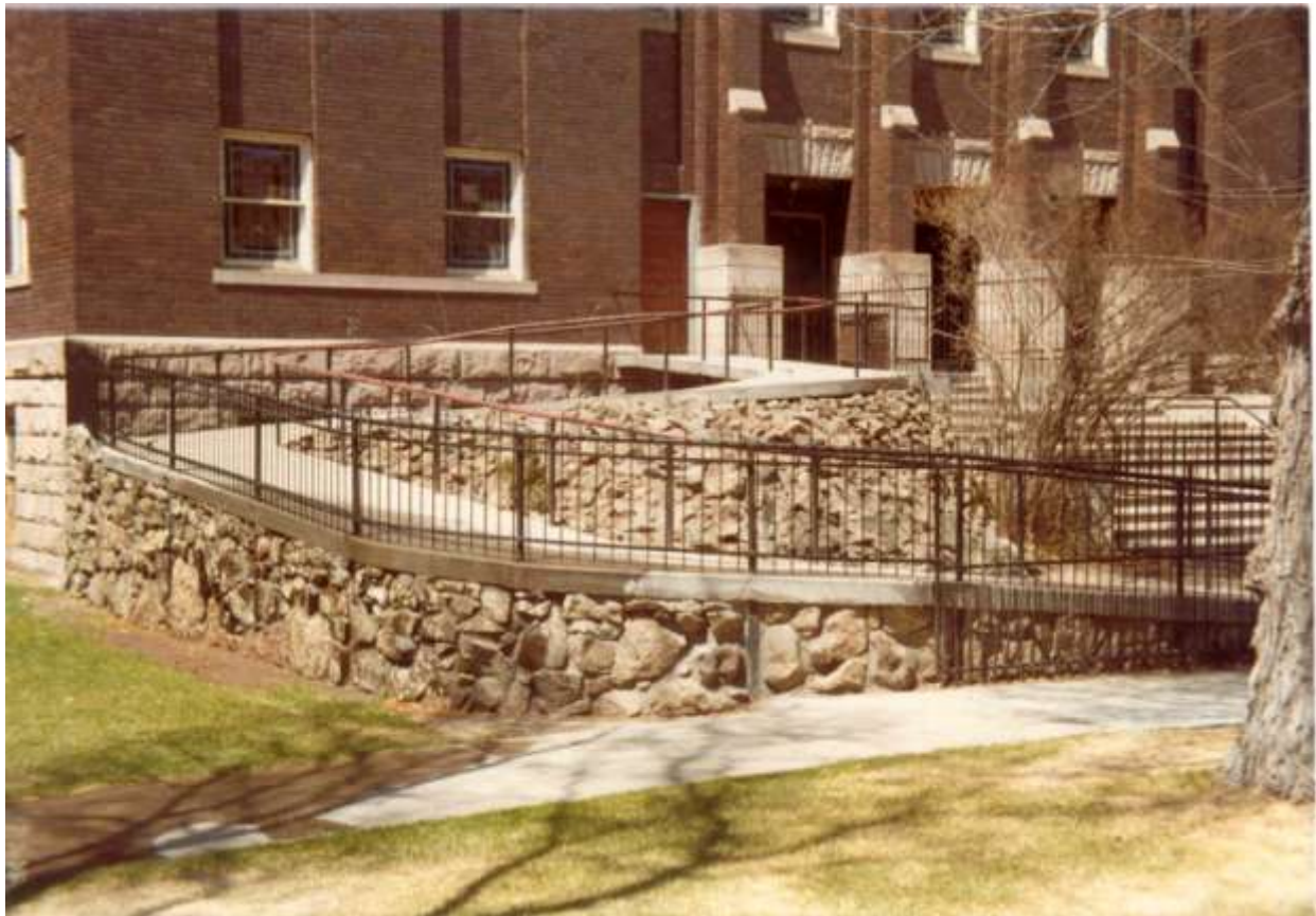
The ramp, a challenge to navigate for even the ambulatory.
