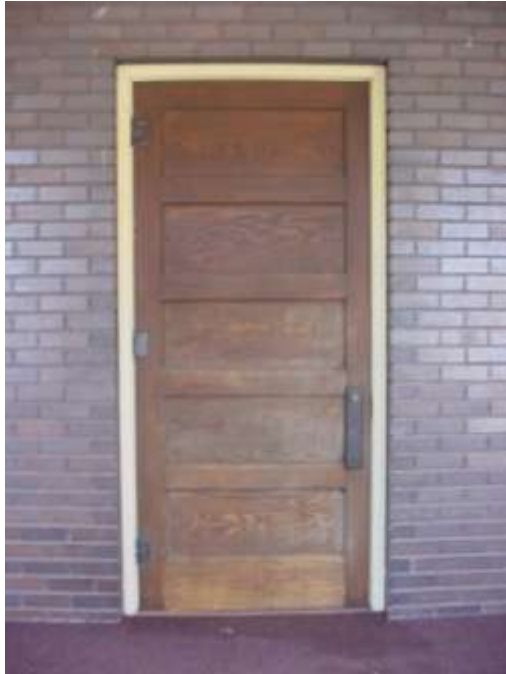
Main entry door at east face.
