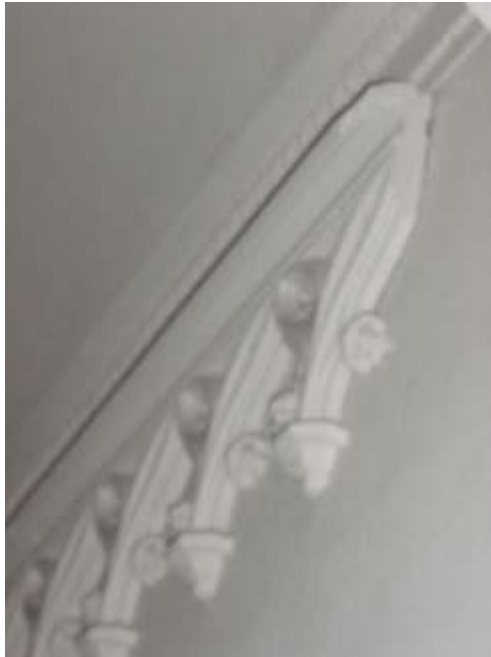
Detail at plaster gothic tracery
