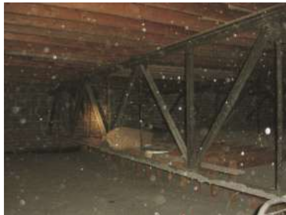
Above and above right: Steel trusses in attic. White flecks are insulation fabric
