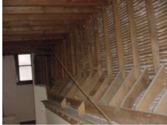
Framing above stage.
