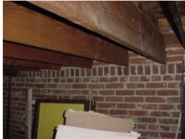
Composite beam in storage room below chancel. 2 x 12 joists below chancel.
