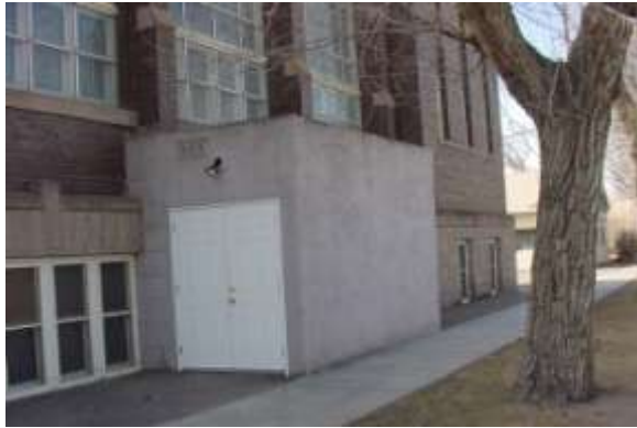
Exterior of entry vestibule.
