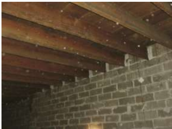
Roof joists in attic
