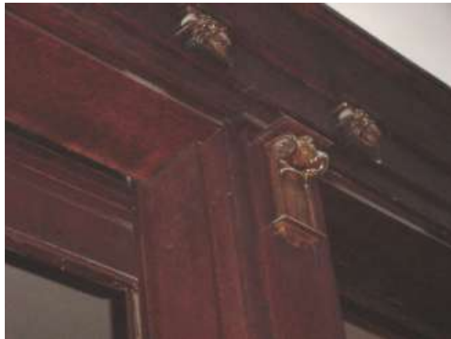
Below: Wood brackets and corbels at overhead partition wall
