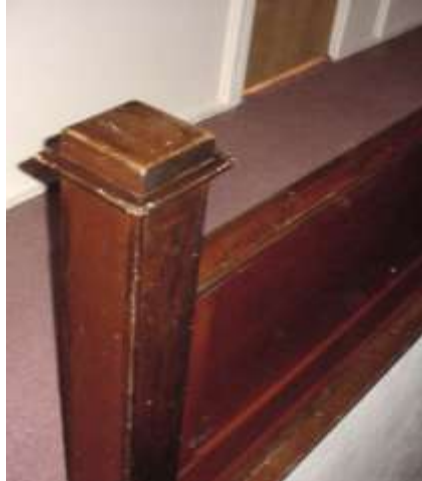
Mezzanine newel and guardrail (overlooking assembly hall)
