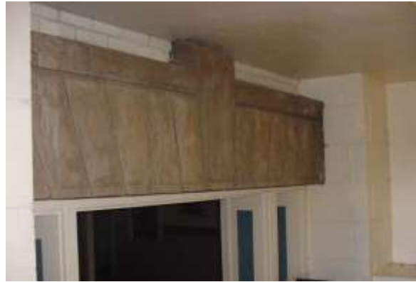
Arch at entry vestibule interior, looking in to dining room
