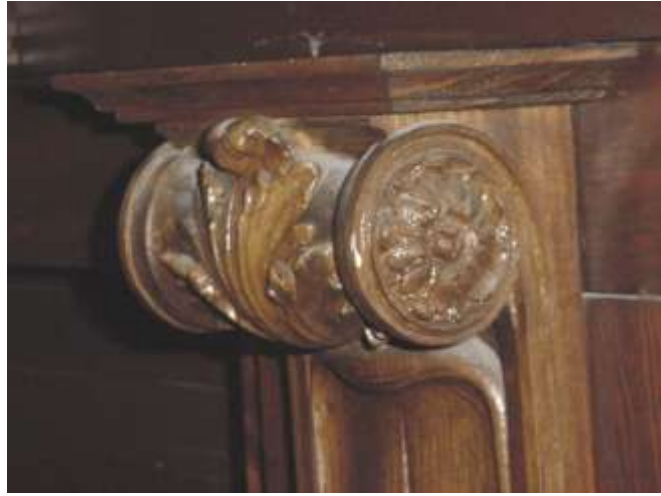
Left: Wood Corinthian capital Below: Detail of wood bracket at overhead partition.
