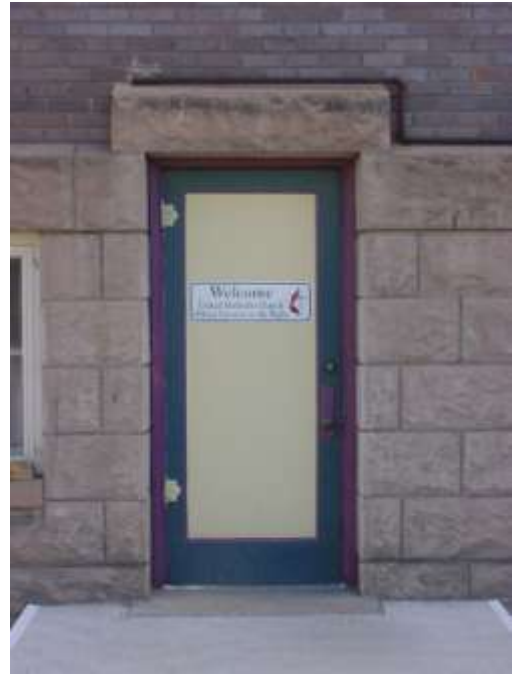
Entry door at west face.
