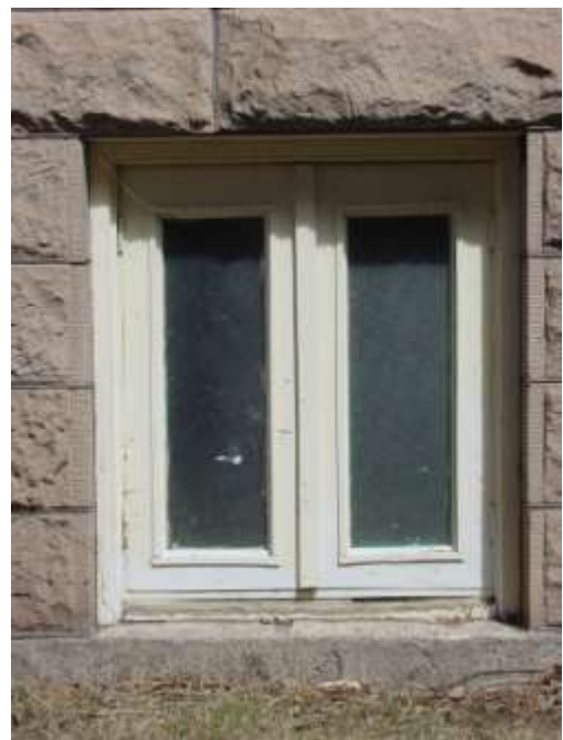
Basement casement window.
