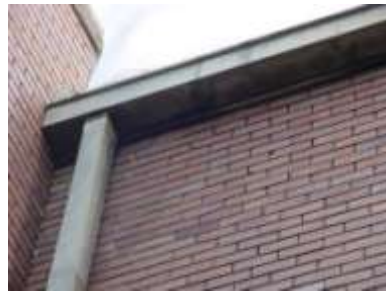
Gutter and leader at west side of south elevation.
