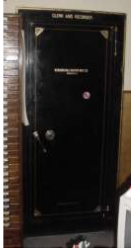
Vault door, exterior. Vault door with cylinder lock.
