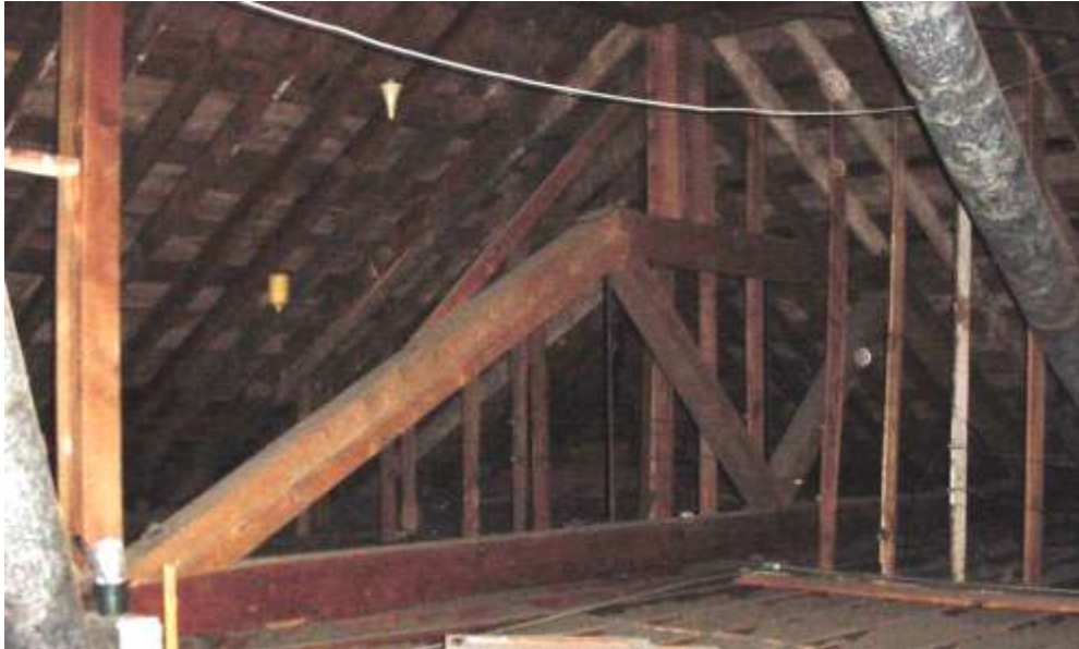
One of four 8x10 construction girder roof trusses. Note vertical steel tension rods.
