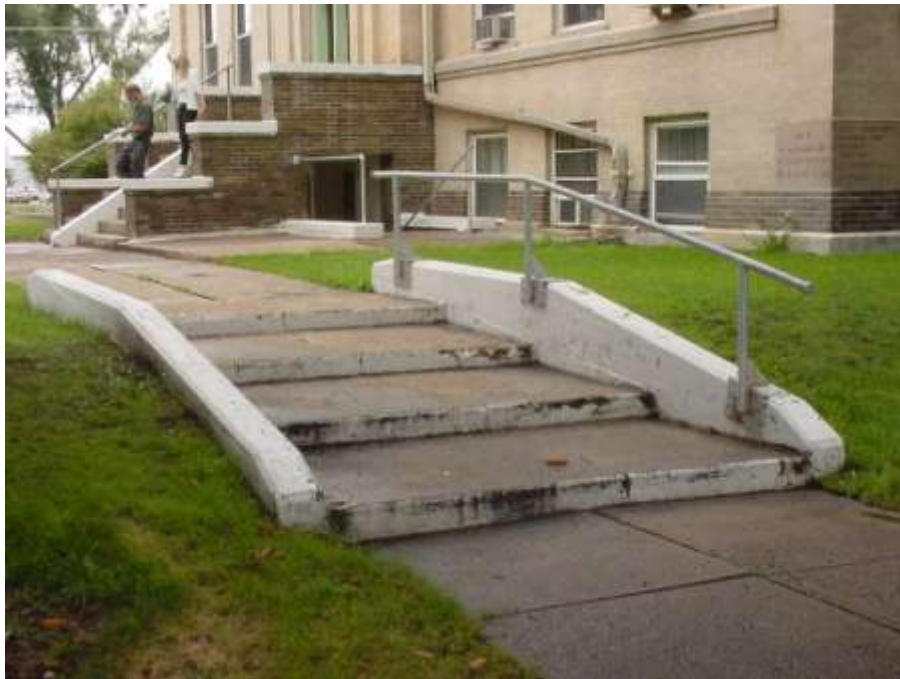
Side (northeast) site stair.
