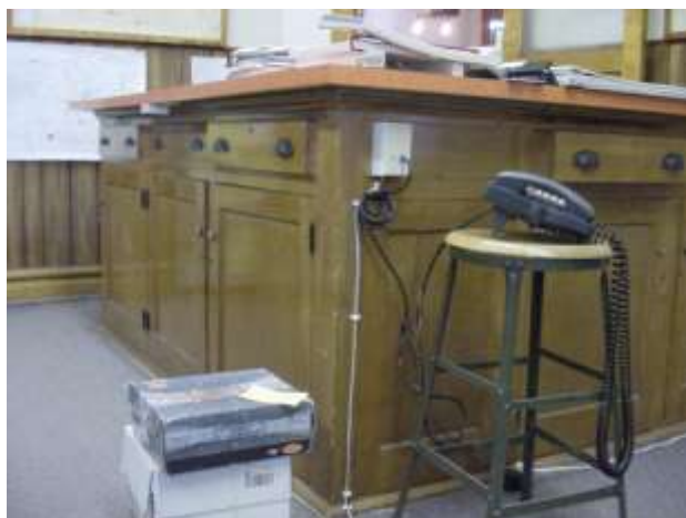
Original desk and counter in clerk's office. Note non-original plywood wainscot, which should be removed.
