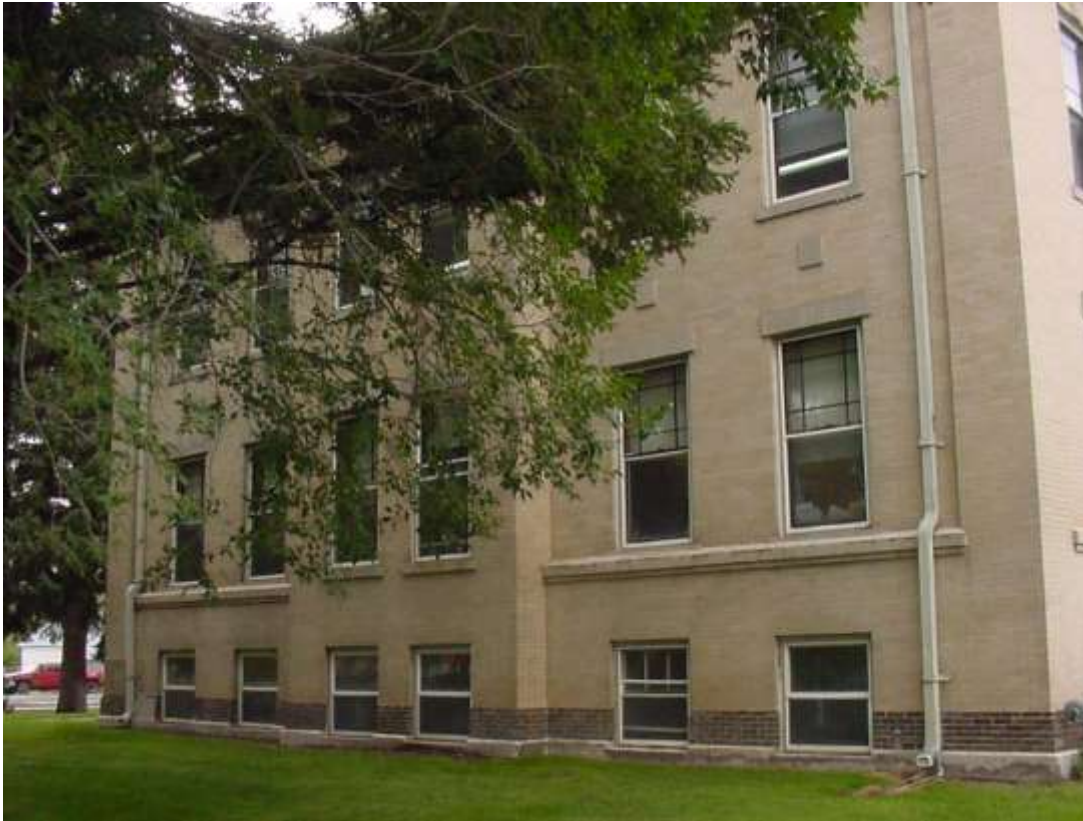
Saguache County Courthouse, side (north) elevation, partially visible through trees
