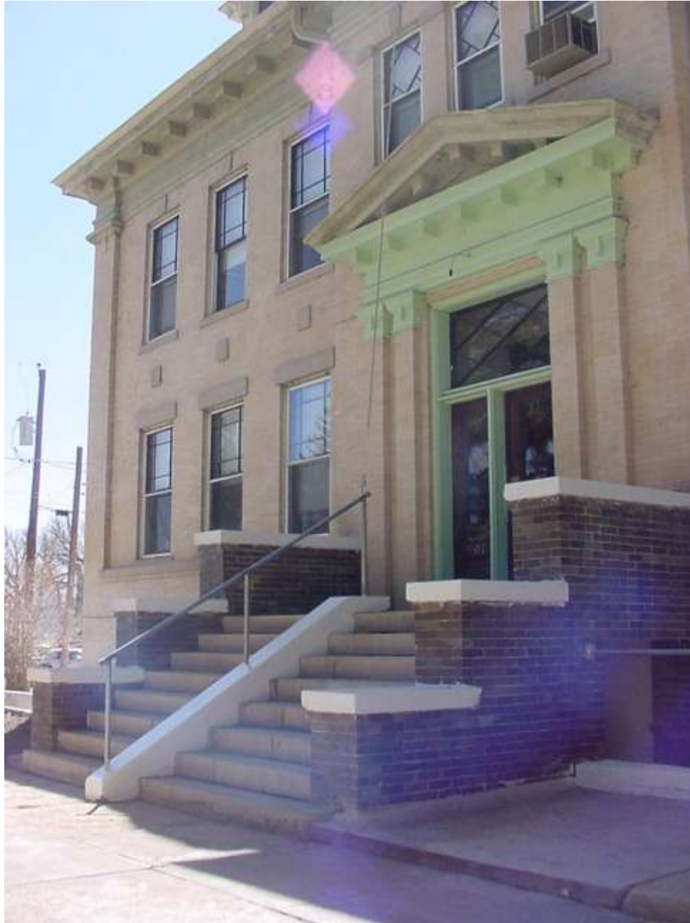
Entry photo, showing front stair.
