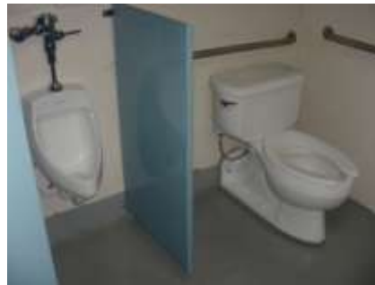
Accessible restroom fixtures
