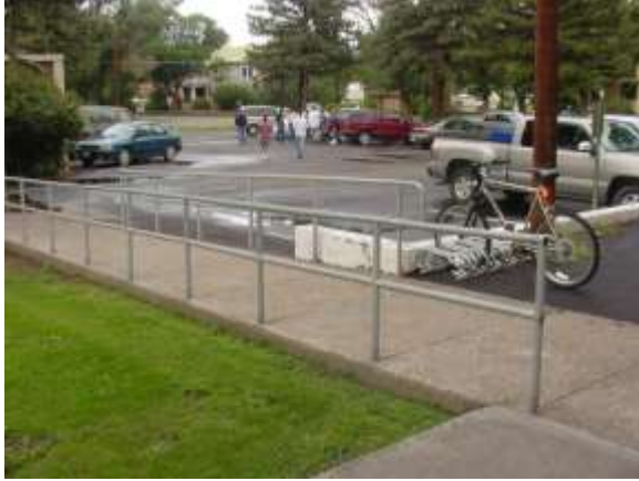
Walk from west entry towards the west. Note slight slope (<1:20) and handrails.
