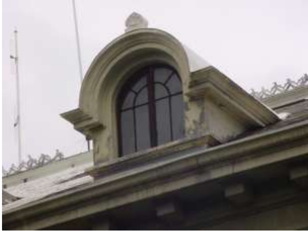
Dormer exterior, with galvanized sheet metal detailing.
