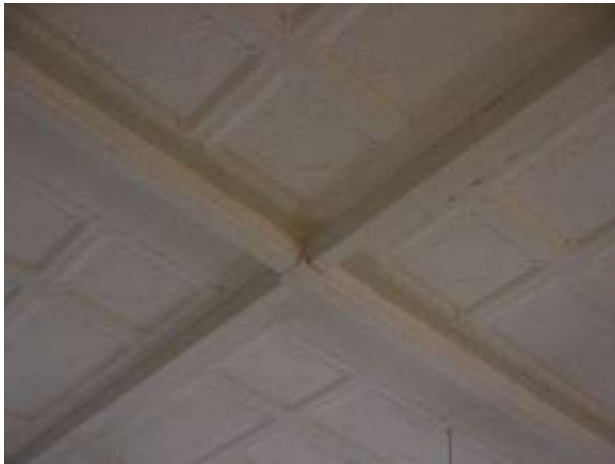
Tin ceiling in courtroom.
