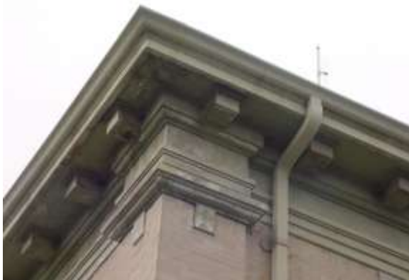
Pilaster capitol, and cornice with dentils above.
