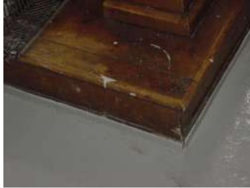
Stair with separating edge trim at lower level.
