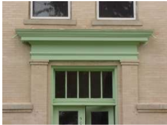
Back (west) entry cornice
