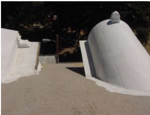
Above: View of galvanized iron dormer
