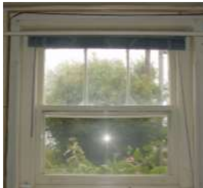
Lower level window, interior
