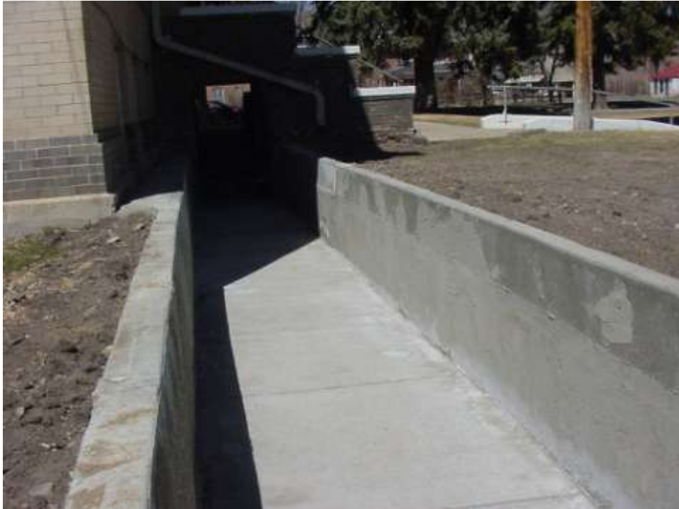
Sloped concrete walk on east elevation, constructed by county crew in 2002, with retaining walls on each side.
