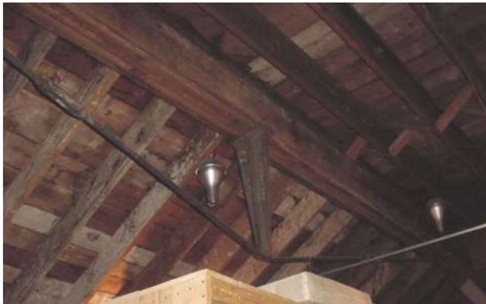
Hog chain trusses in attic, supporting edge of flat roof and rafters.
