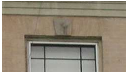
Below: Upper level window brick jack arch with brick key plastered with cement.
