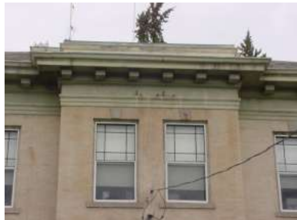
Pilaster capitol, and cornice with dentils above.
