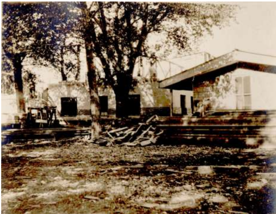
Start of foundation of new courthouse. Otto Mears' residence to right.
