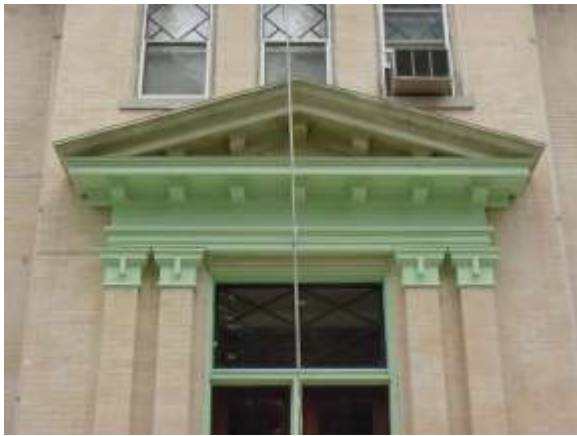
Front (east) entry pediment
