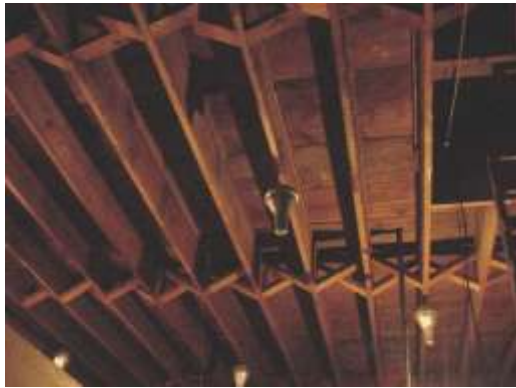
2x12 deck joists with 2x4 bridging
