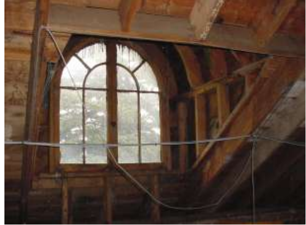
Dormer, interior, showing 2x6 wood framing.
