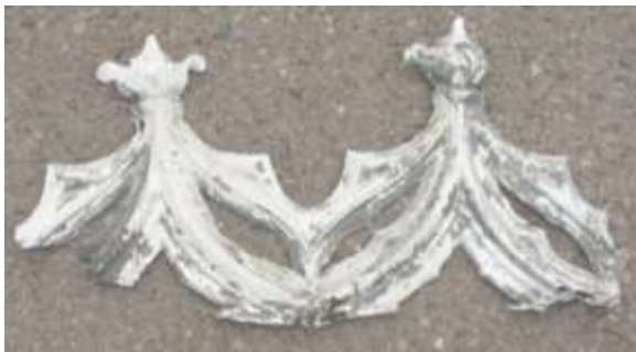
Portion of original iron cresting.
