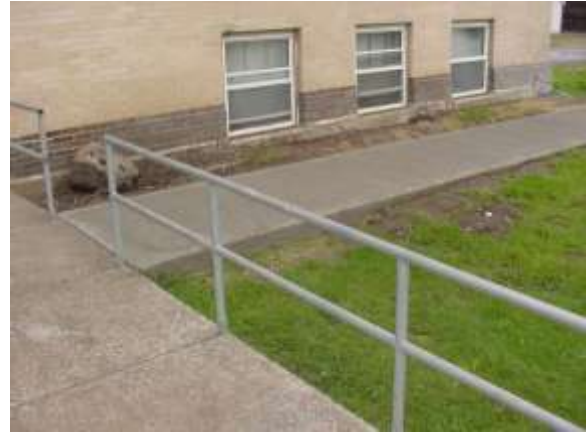
Walk from west entry towards the south.
