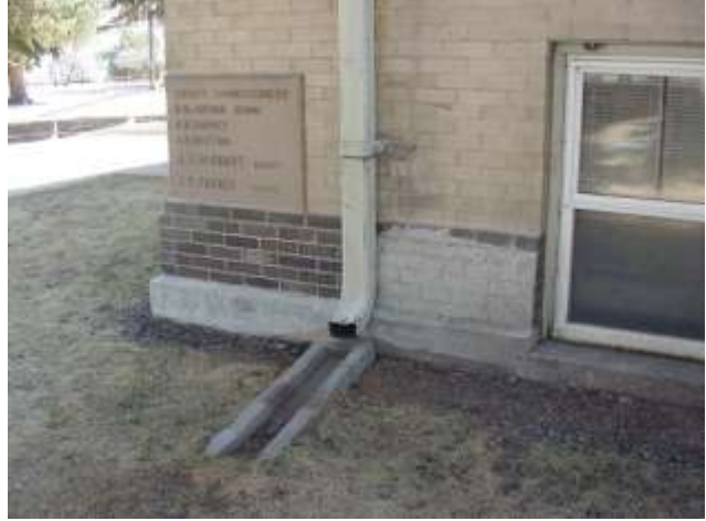
Painted brick, to right of downspout.
