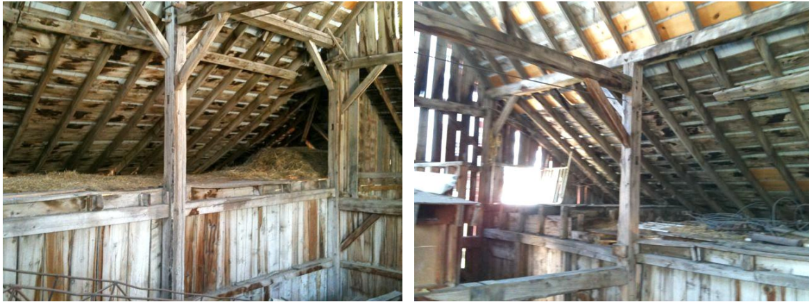
Interior photos of barn, showing steel tension rods. (Packer, 2010).
