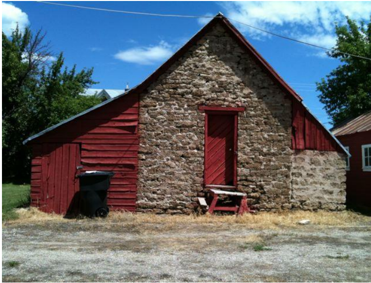
Granary west elevation. (Packer, 2010).
