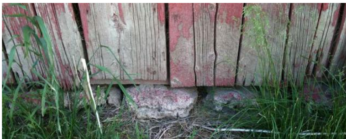
Barn foundation (cropped). (Packer, 2010).
