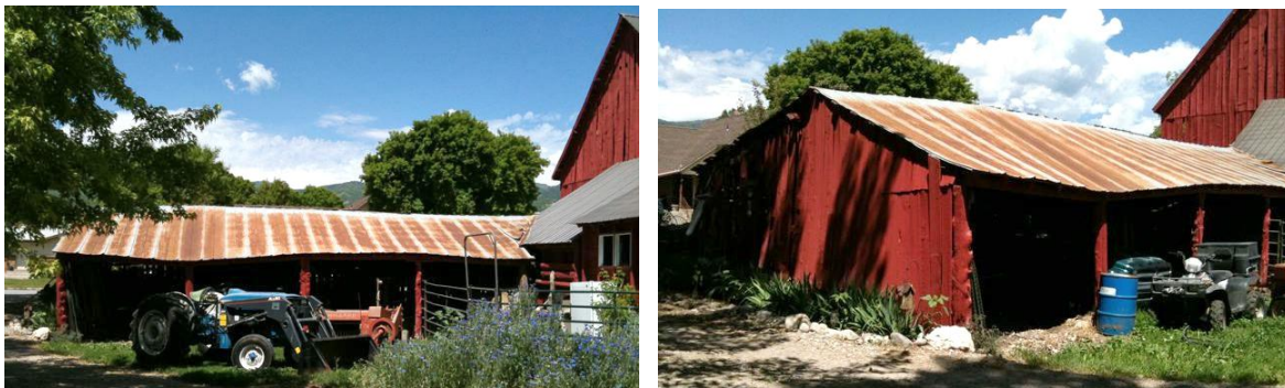
South barn addition. (Packer, 2010).
